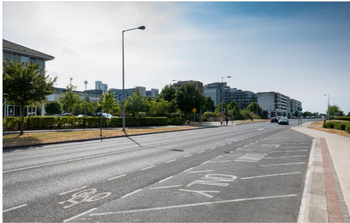
VIEW 2 – View from Blackthorn Avenue looking Southwest
