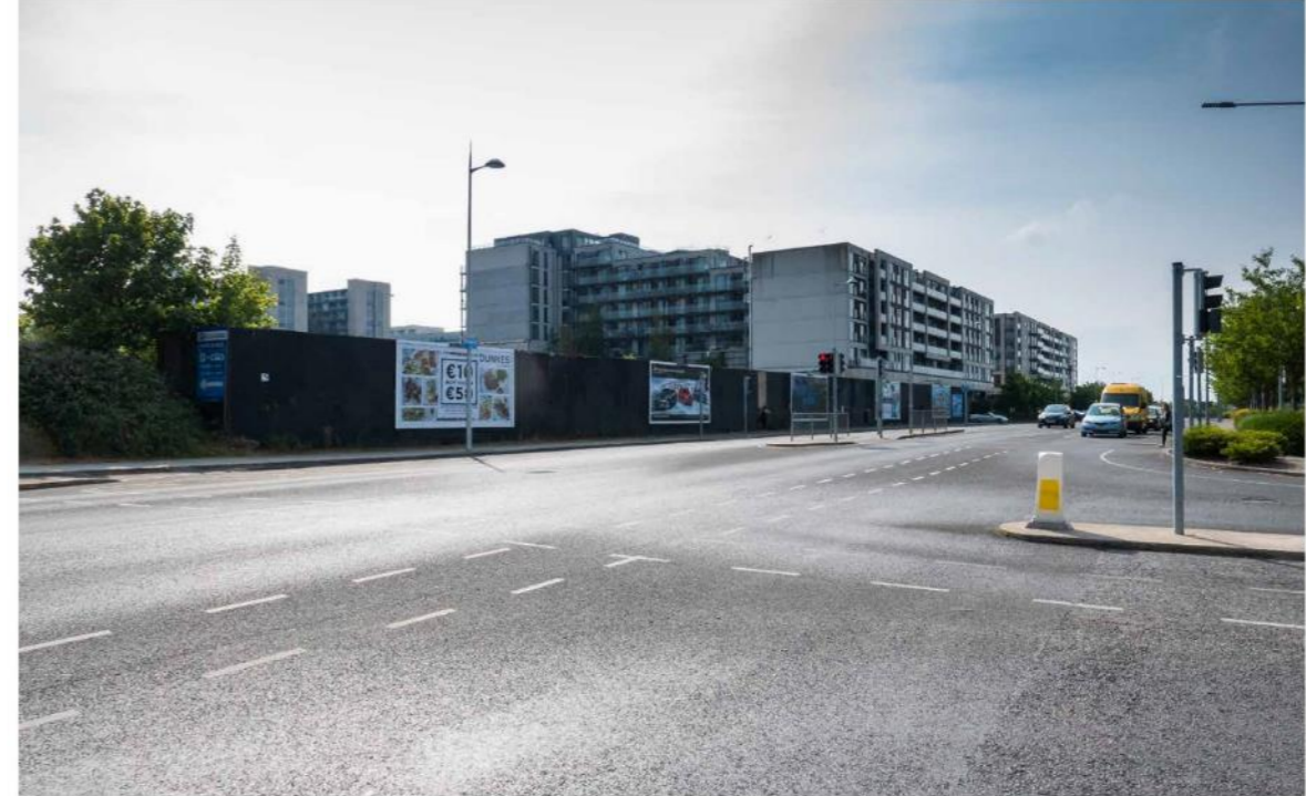
VIEW 3 – View from junction of Blackthorn Avenue & St Raphaela's Road looking Southwest
