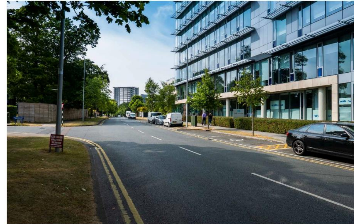
VIEW 1 – Carmenhall Road looking West
